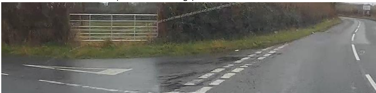
R5.23a - Condition Score 40 (Junction markings)
