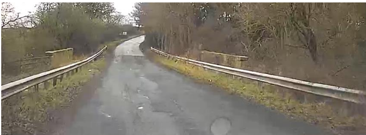
R3.24 Condition score 0 (very Poor road surface at water crossing)
