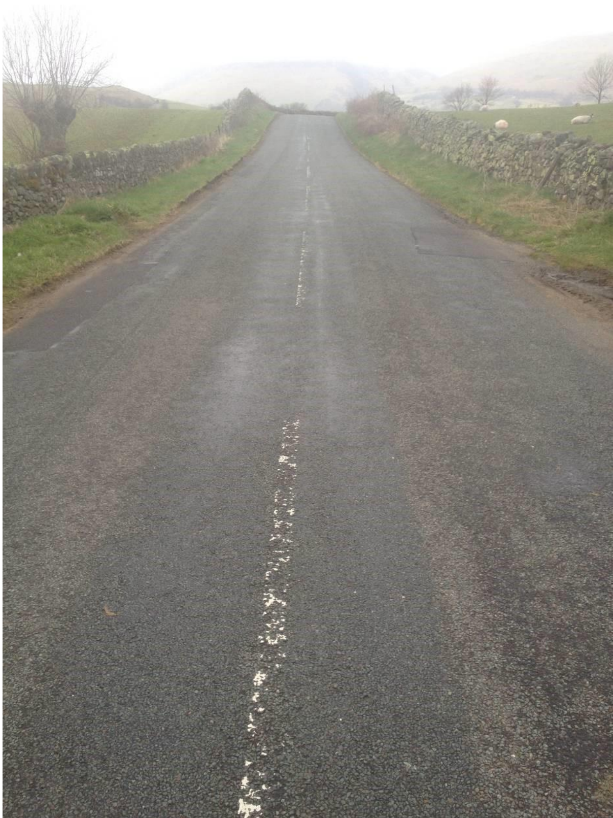
Figure C.14 Condition score 0 – long view
