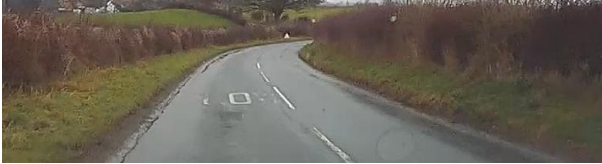
R2.20 - Condition score 0. (no marking approaching junction)
