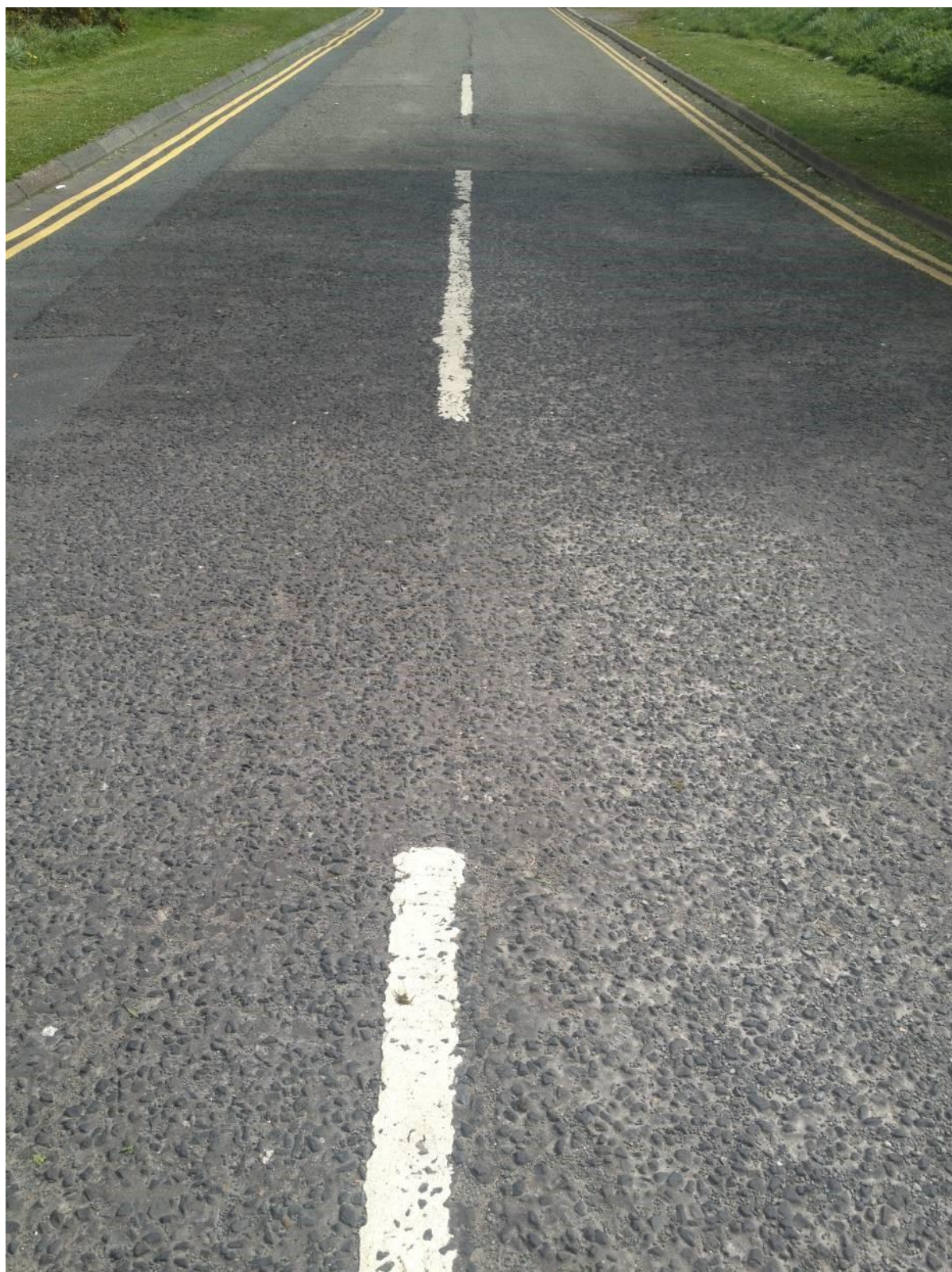
Figure C.10 Condition score 20 – long view
