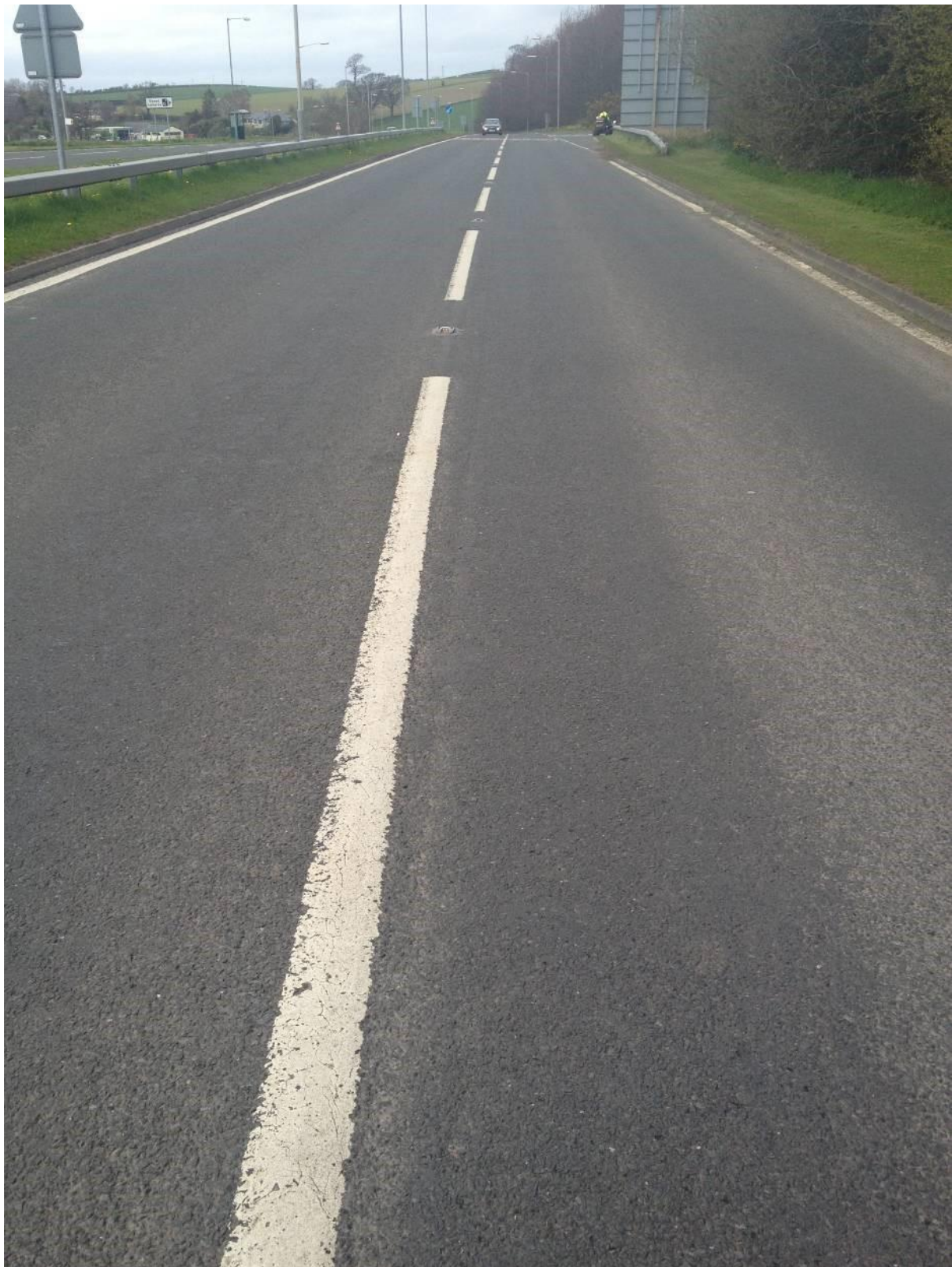
Figure C.7 Condition score 30 – long view
