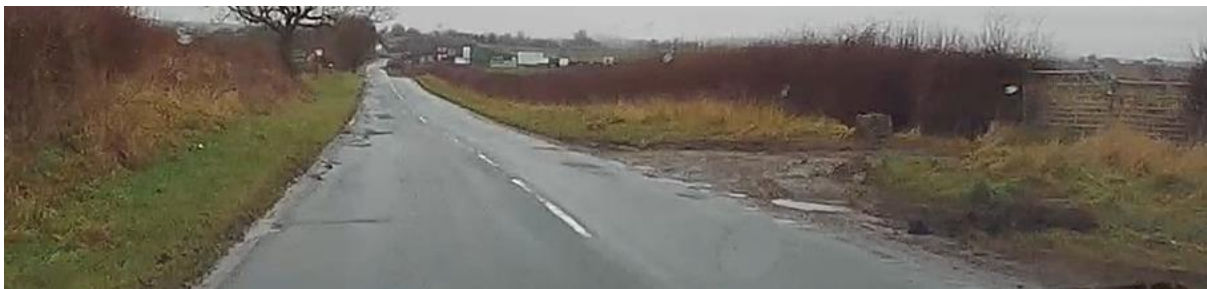
R2.13 - Condition score 10 (Note Lane surface extreme poor condition) forced to use centre of carriageway!
