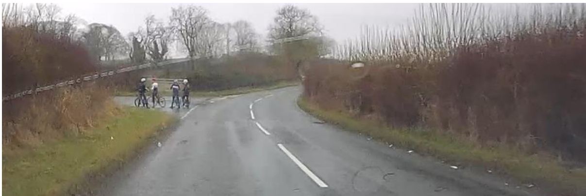
R5.23a - Condition Score 40 (Junction markings)
